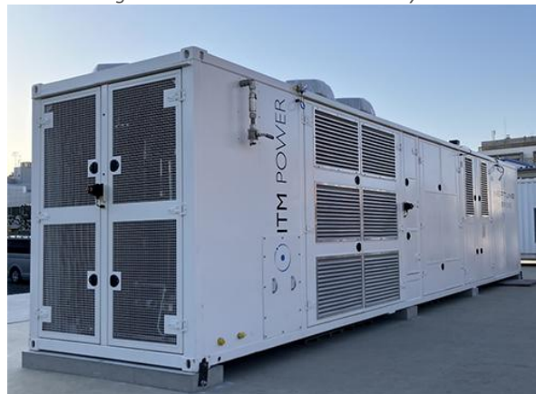
Figure 74 - 1 MW ITM PEM electrolyzer.
