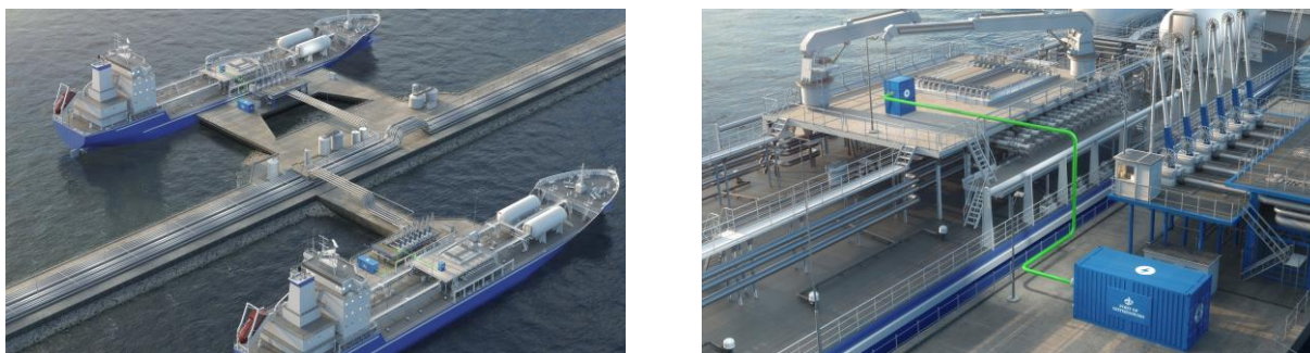
Figure 46 - Example of OPS installation for tankers: The Green Cable project for tankers at the Port of Gothenburg.
