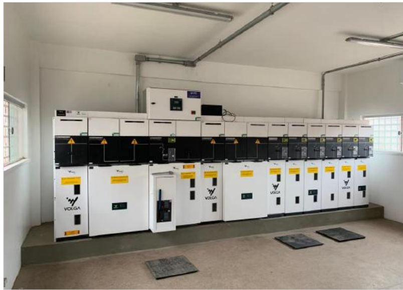
Figure 64 - EMAP medium-voltage panel [6].
