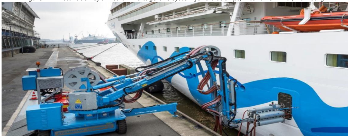
Figure 24 - Installation of a medium-voltage OPS system for cruise ships, Altona Terminal, Hamburg.
